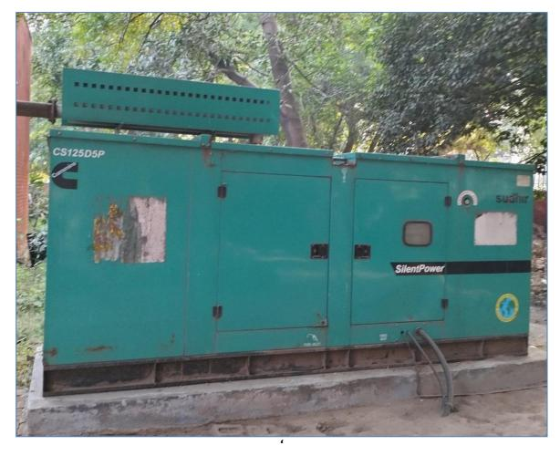
**Observation and Suggestions**:- As per the trial taken during the energy audit the percentage loading of DG set is 61.56% which is ok and specific energy consumption of DG Sets 3.12 KWH/Litre which is satisfactory because as per manufacturer recommendation, best practices for SEC in DG sets range from 3.0 to 3.5 kWh/litre and above.
